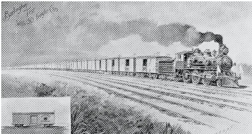
● CB&Q hosted an air-brake trial with 50-car blocks in West Burlington, Iowa, in 1886. The inset shows a boxcar outfitted with a "slideometer" to measure shocks experienced in the last car. Eleutherian Mills Historical Library
