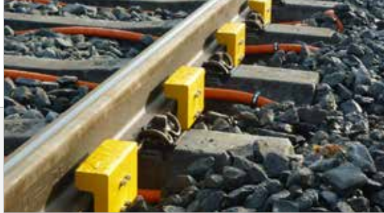
WHEEL CONDITION MONITOR
