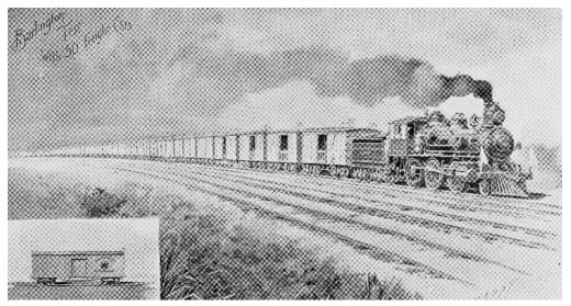
• CB&Q hosted an air-brake trial with 50-car blocks in West Burlington, Iowa, in 1886. The inset shows a boxcar outfitted with a "slideometer" to measure shocks experienced in the last car. Eleutherian Mills Historical Library
